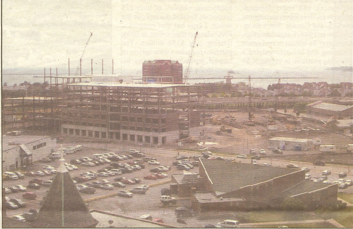
Construction of the new BlueCross/BlueShield of Western New York headquarters, Buffalo
